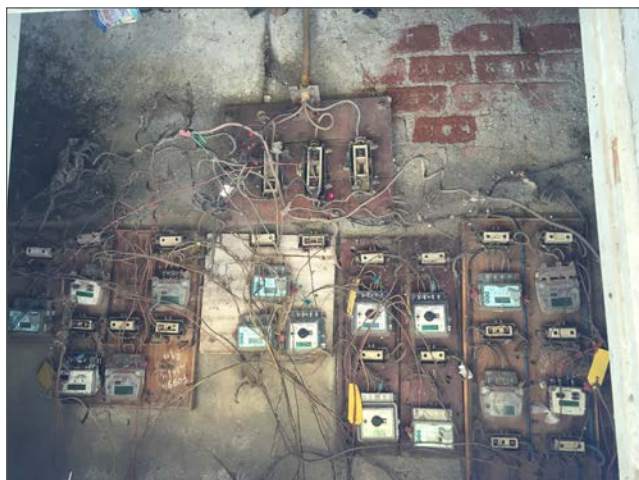
FIGURE 14: ELECTRICITY CONNECTIONS INCLUDING INDIVIDUAL AND “SHARED” CONNECTIONS IN A SLUM IN MUMBAI
