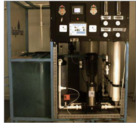
Decentralized water plant by Sarvajal
