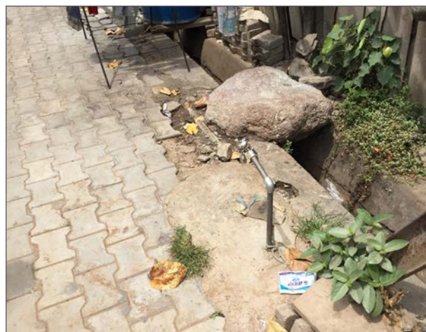
FIGURE 18: OPEN DRAINAGE ALONGSIDE A WATER PIPE NETWORK IN A NOTIFIED SLUM IN PUNE
